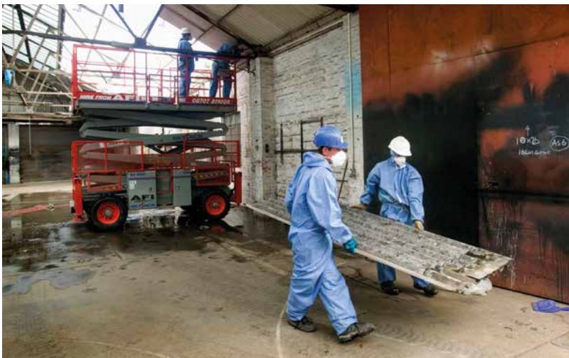
Asbestos is removed from a factory roof in Bristol © Paul Box/reportdigital.co.uk
